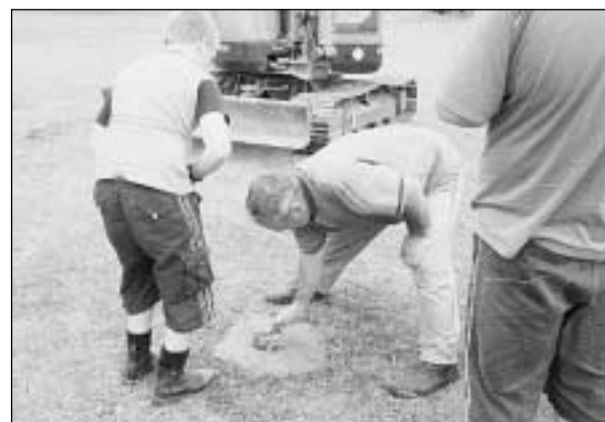
Installation of the chopping bases.
